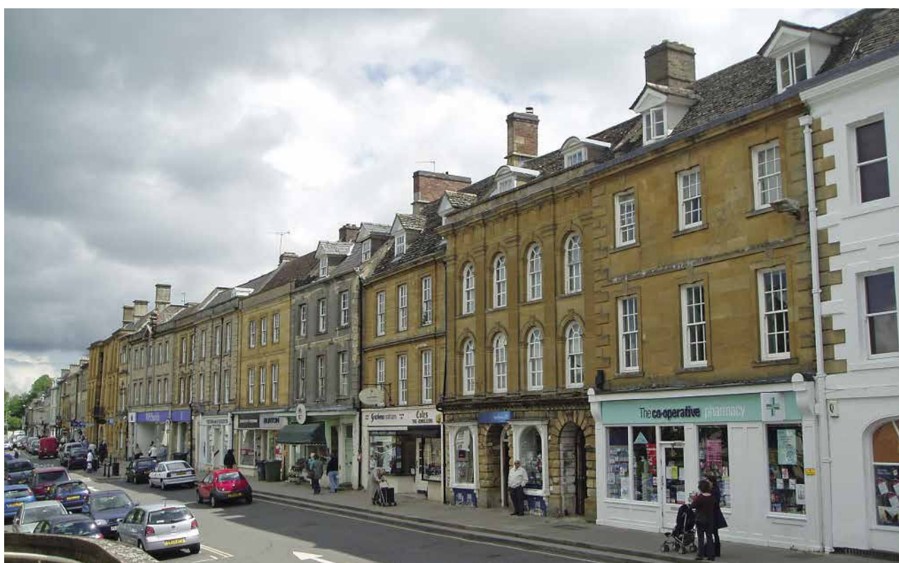
Figure 16: 25 & 24 High Street, Chipping Norton, Market Place Top Side
