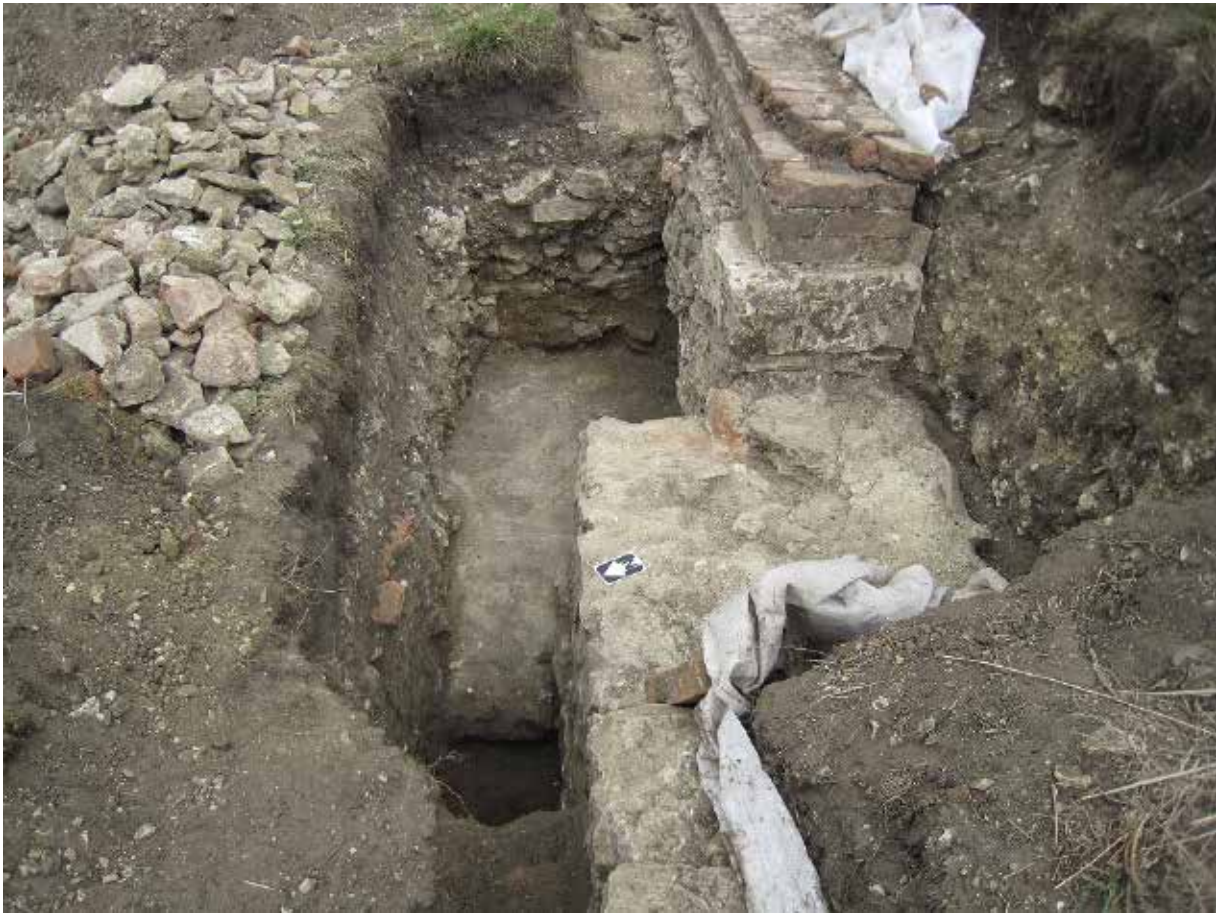
Figure 24: Ascott Park, In the foreground is the 0.85m wide house south wall. Beyond it is the north-east terrace retaining wall
