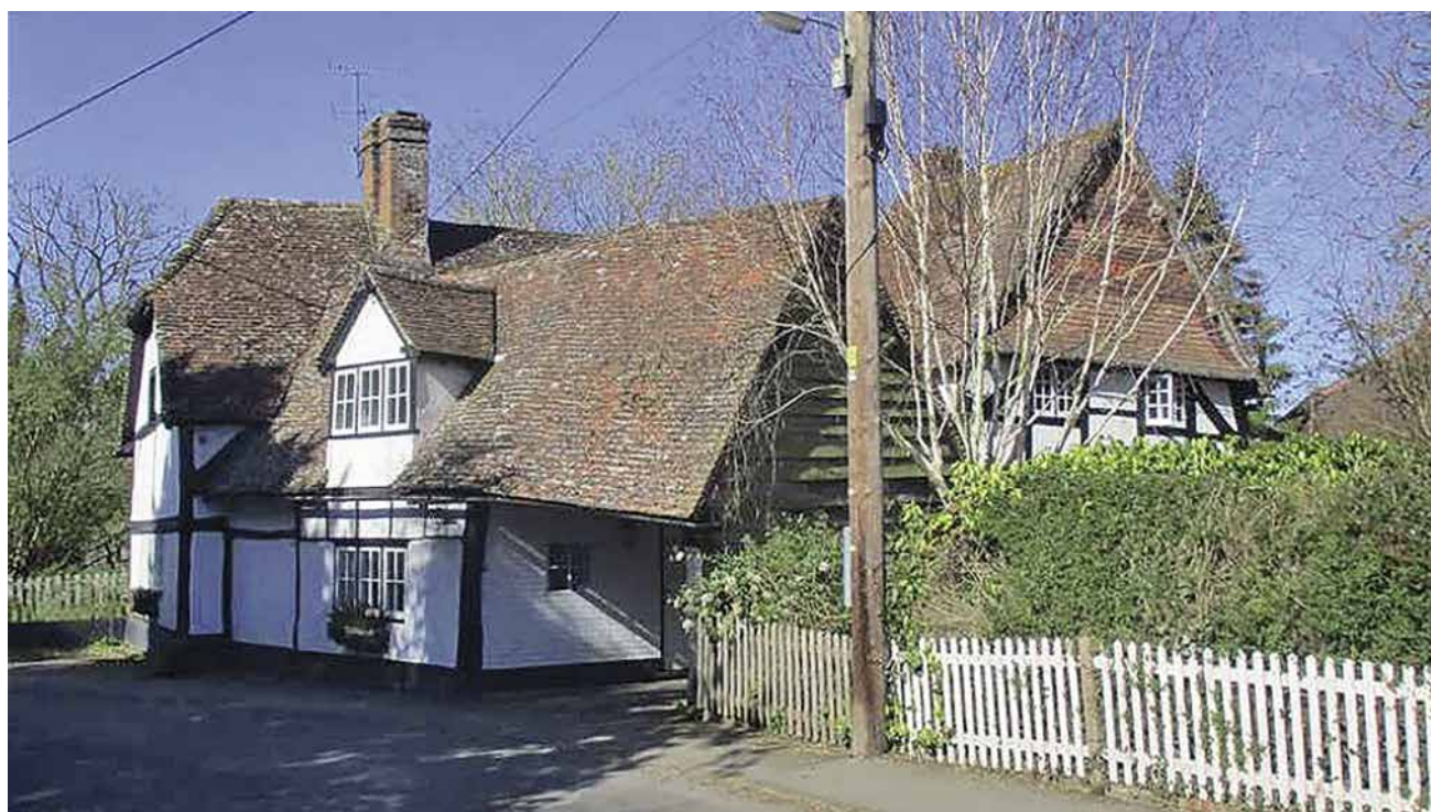
Figure 11: The Gables, East Hagbourne
