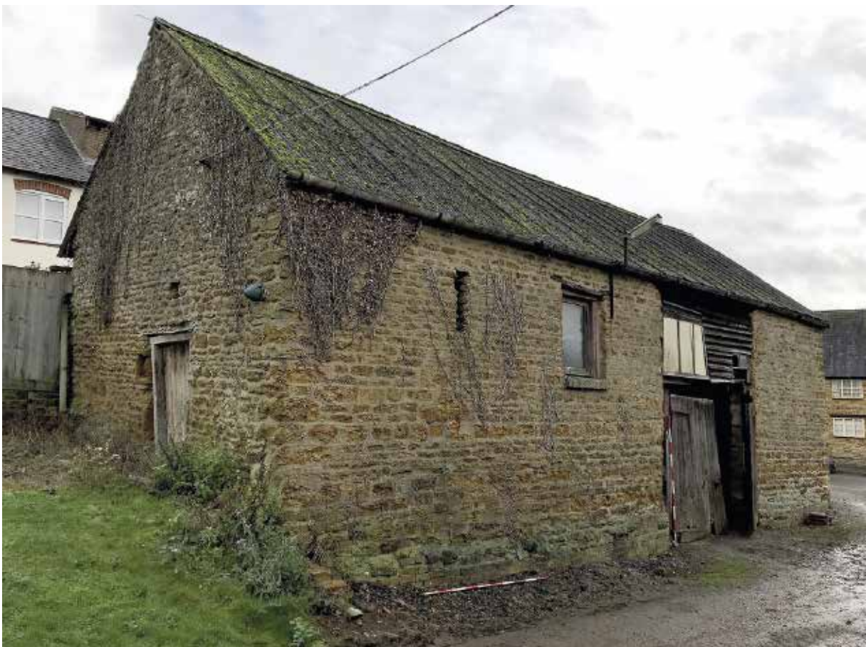
Figure 15: Earls Barton, bank barn
