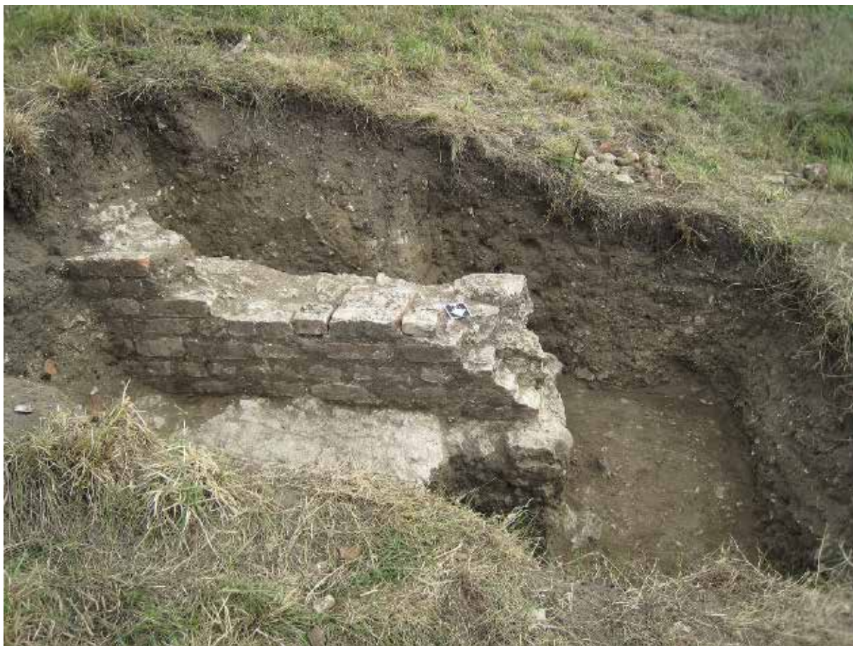
Figure 22: Ascott Park, The western end of the north-west terrace retaining wall looking south
