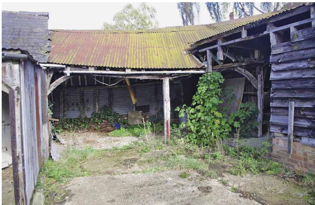
Figure 16: Outbuildings at 16 Main Street, Mursley, 1m scale (photograph by Gerwyn Richards)
